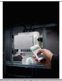
05: The eSchell water management system allows for the networked operation of Schell sink, shower, WC and urinal valves and can be integrated into primary central building control system networks.
